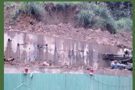
Remedial works, Nangang retaining wall, Taiwan
