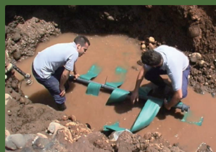
Seawater Desalination plant, Spain
