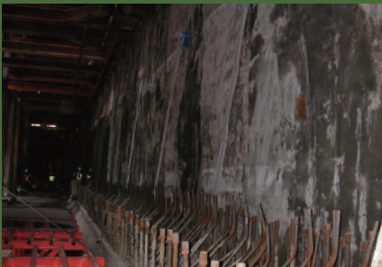
Kaohsiung Mass Rapid Transit Tunnel Drainage, Taiwan
