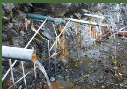
Community Small water treatment, Taiwan Hualien
